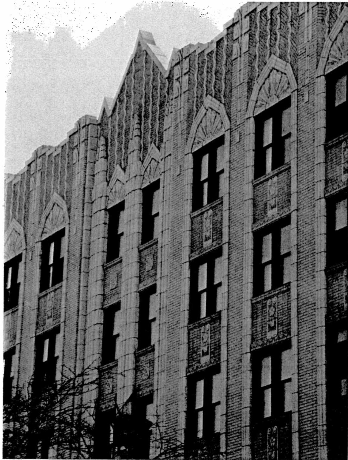
Above: The combination of the continuous vertical piers with the understated spandrel panels lends the Union Park Hotel a strong vertical emphasis, another important trait of the Art Deco style.
